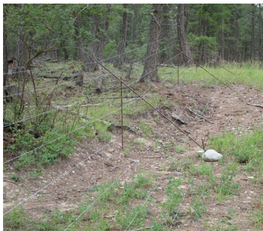
Slant fence design from Grave Creek, Montana
